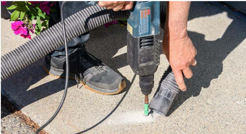
**7** Hammer the concrete anchors into the clean drilled holes so they are slightly below flush with the surface. This is easiest with a sacrificial bolt.
