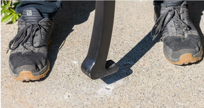
**10** Bolt the bench to the anchors with the supplied bolts and washers.
