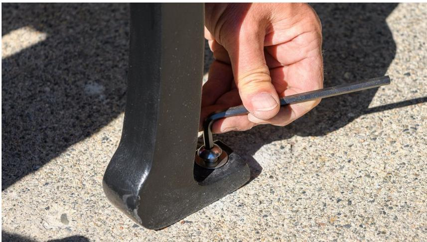
**11** Optional. For theft resistance, fill in the bolt heads with silicone and paint the tops of the fasteners with a paint pen to match the colour of the frame.
