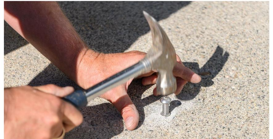
**8** Fix the anchors in place with the supplied set tool and a hammer to expand the base of the anchors and permanently secure them to the pad.
