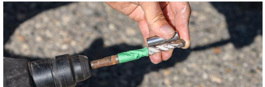
**5** Drill all holes to the depth indicated by the tape or marker applied to the drill in step 4. Holes must be vertical to properly anchor the bench.
